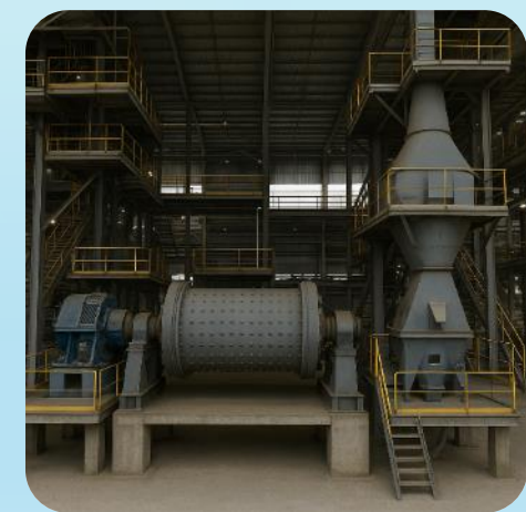
Cement mill retrofit
